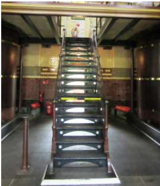
Stairs to Upper Floors
