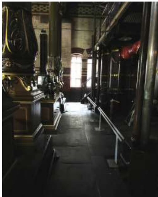
Route to Switch Room
